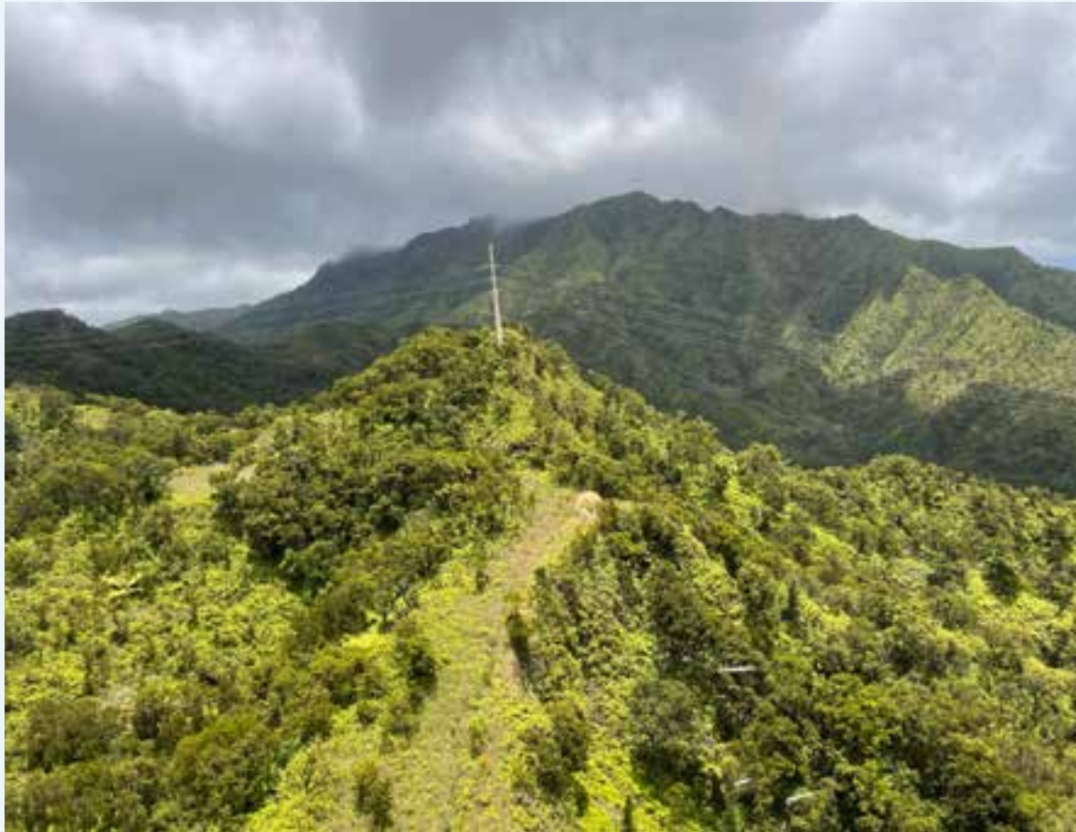
Figure 36. Powerline collision area, Kaua'i, Hawaii. Photo: André Raine.
